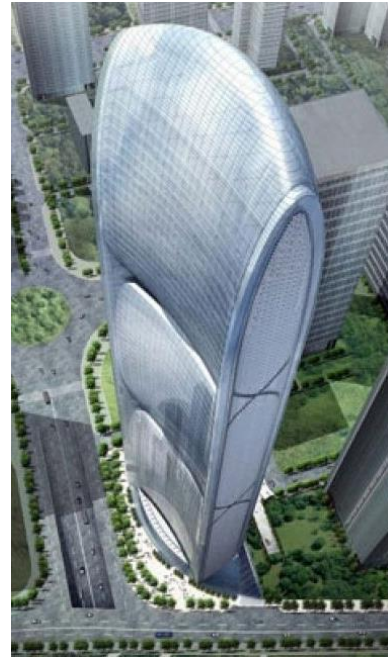
Fig. 14. Zero-energy skyscraper «Pearl River Tower» [23] (spiral "wind vents" are visible on the right side of the house, solar panels are on the facade)
